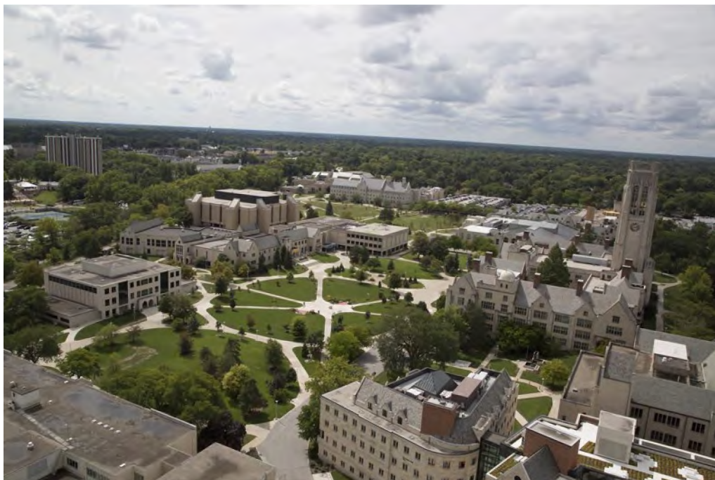
Aerial View of the Main Campus
