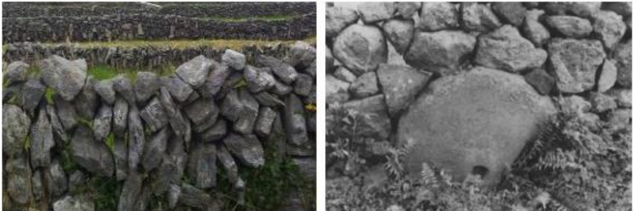
Figure 47-2: Dry (mortar-less) stone wall construction is ubiquitous in Western Ireland (left) and on Jeju Island (right).
