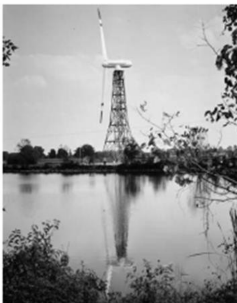
Mod-0 100kW Experimental Wind Turbine in Sandusky, Ohio
