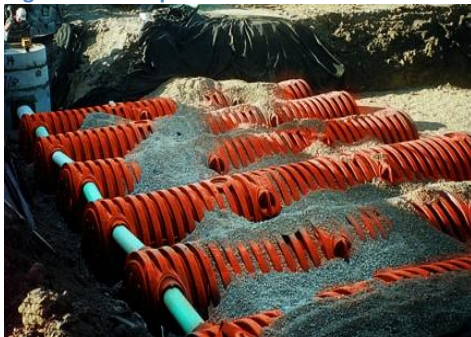
Figure 23: Group installation of storm chamber
