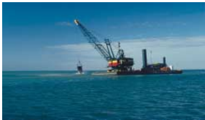
The management of eroded sediment is a costly business.
