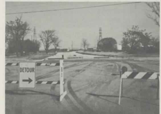
Street re-location and paving
