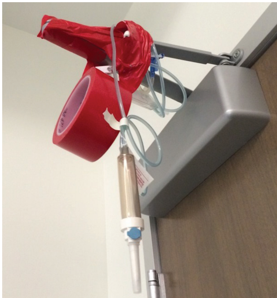
Students used a variety of medical supplies on hand to immobilize the automatic door-closer hinge to bar entry.
