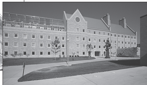
Wolfe Hall was under construction in 1996 and completed in 1997.
