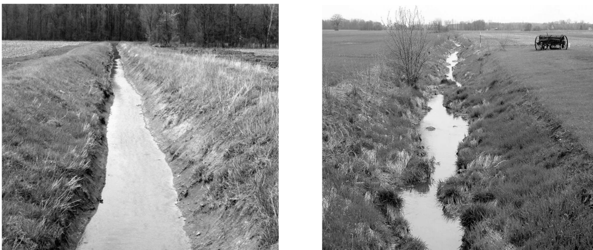
Figure 1: Boyd Feasel ditch, Seneca County (Ohio) in 2008. The left panel shows the ditch North of County Road 36 that was dredged in 2007. The right panel shows the same ditch, dredged pre-2002, South of CR36.
