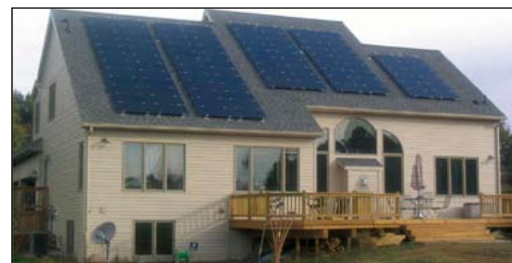
Thin-film solar panels were installed in the roof of Dr. Alvin and Mary Compaan's new house.
