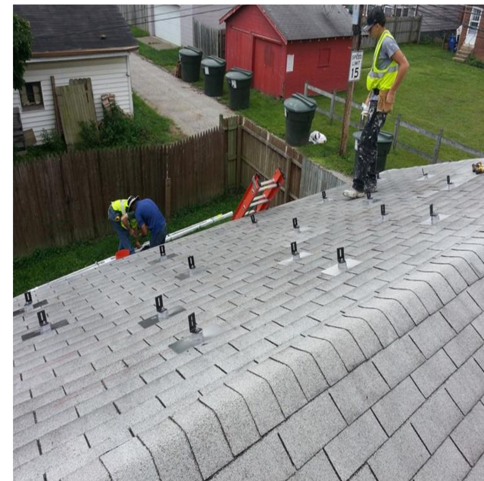
Flashing & L-Foot Located First
