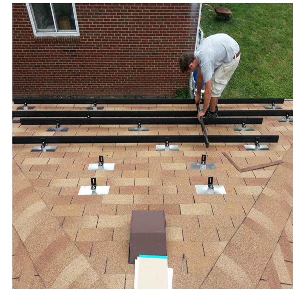
Level Rails are Critical for Aesthetics
