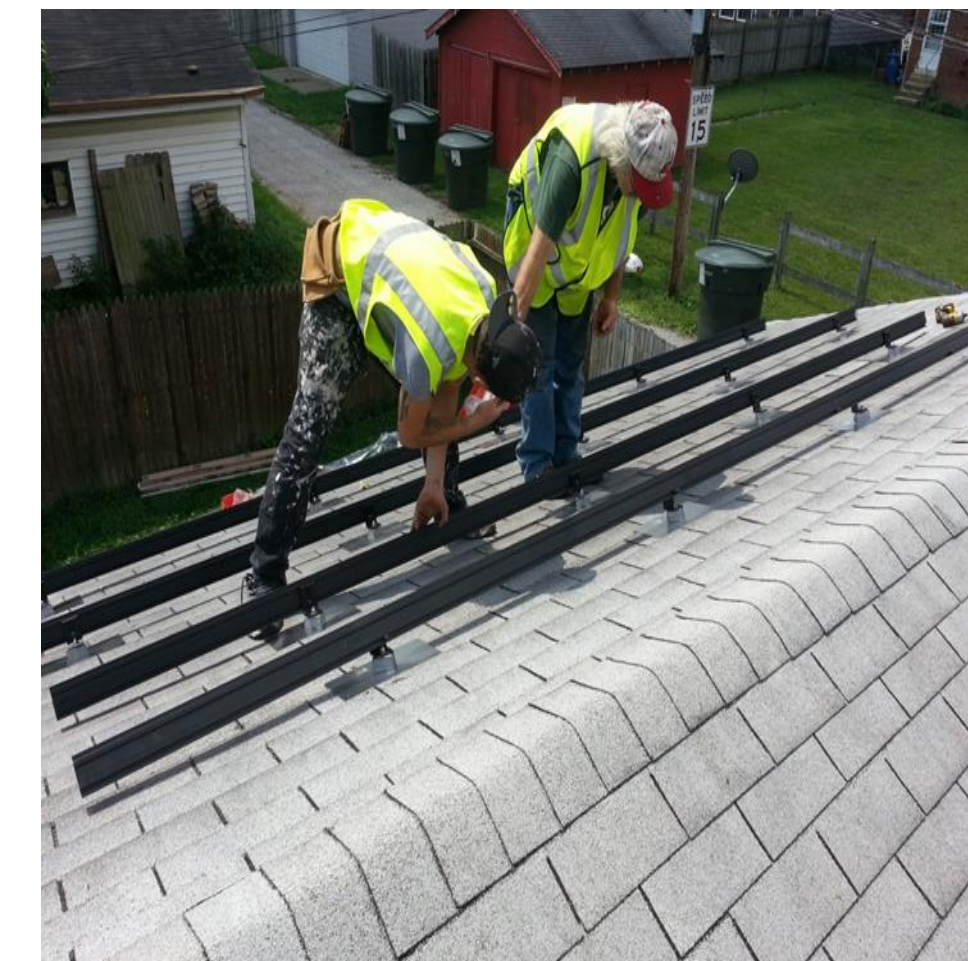
Two Rails Connected to Each Panel Row
