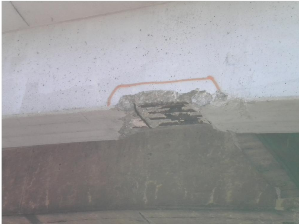
Fig. 1. Damage Caused by Overheight Vehicle Collision
