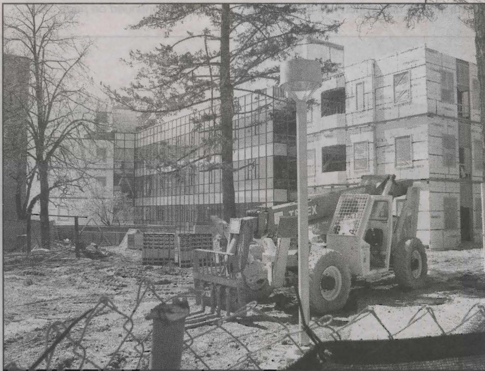
Construction in progress on UT's Savage & Associates Complex for Business Learning and Engagement, set to open later this year
