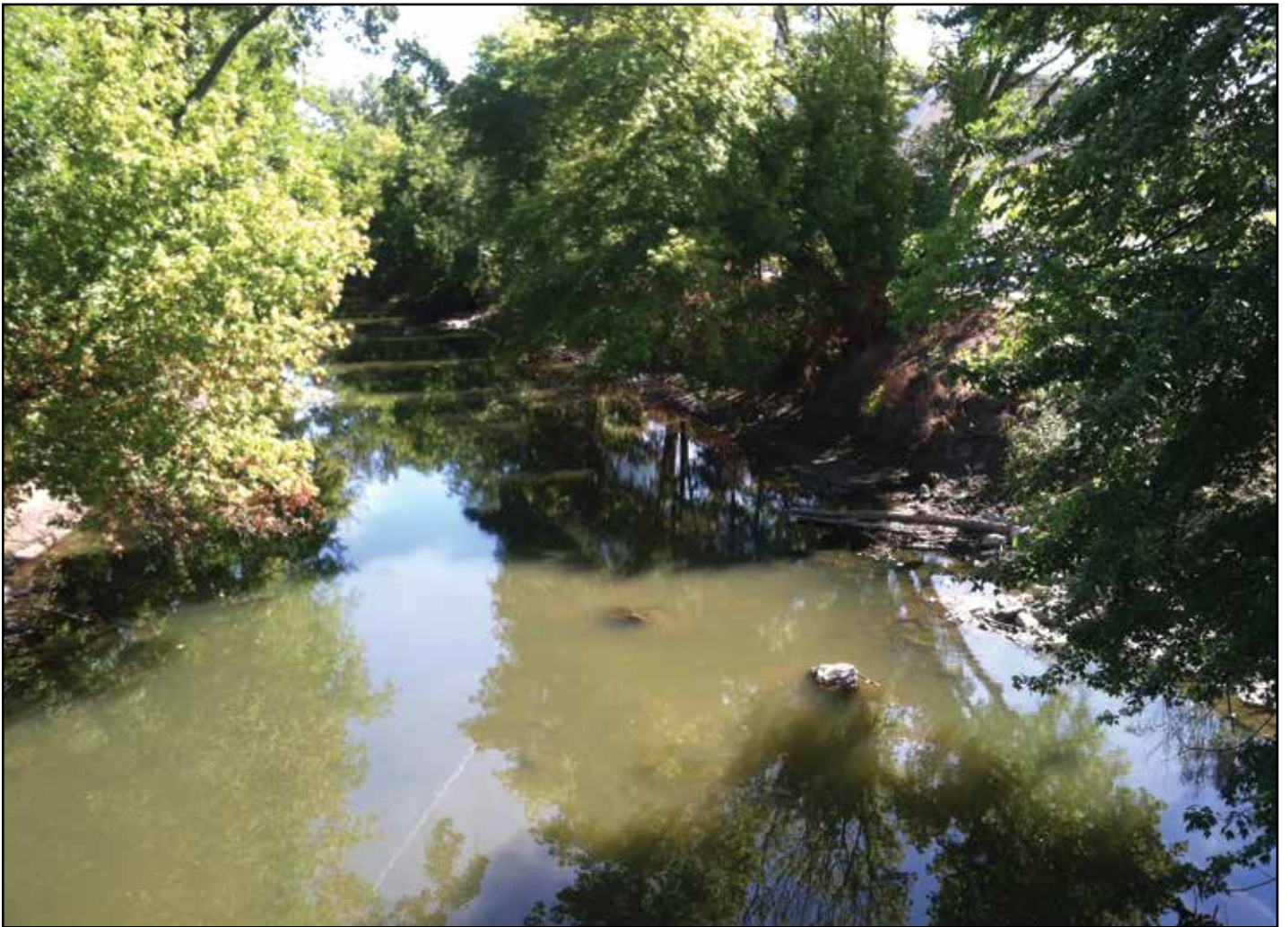
Reach 5 post construction view of hydraulic cover stones and bendway wier with locked log.
