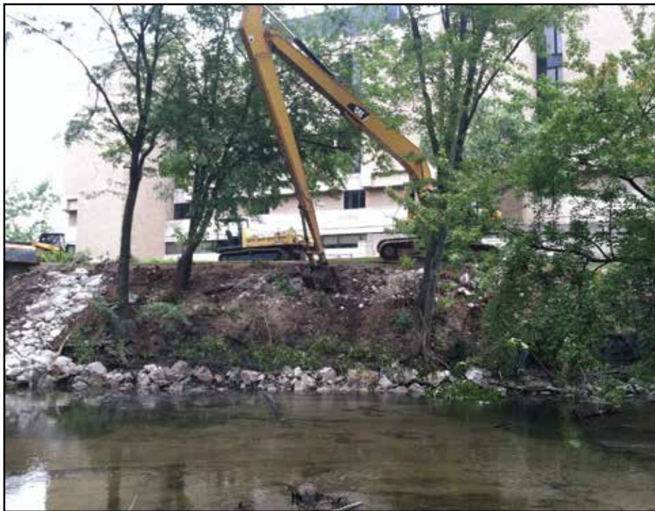
Construction of longitudinal toe protection structure.
