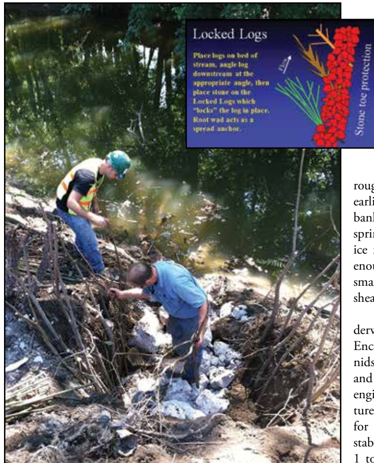
Installation of live stakes in locked log feature.
