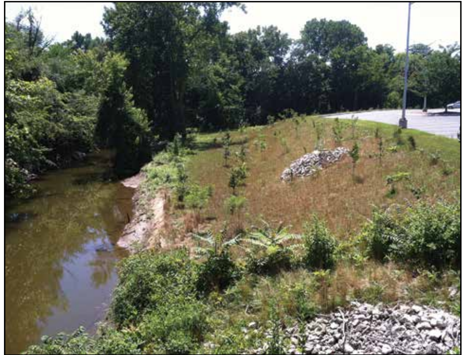
Cutbank feature in Reach 1 in the summer of 2013, one year post construction.
