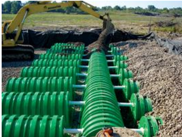
Figure 4: Underground Detention Pipe System
