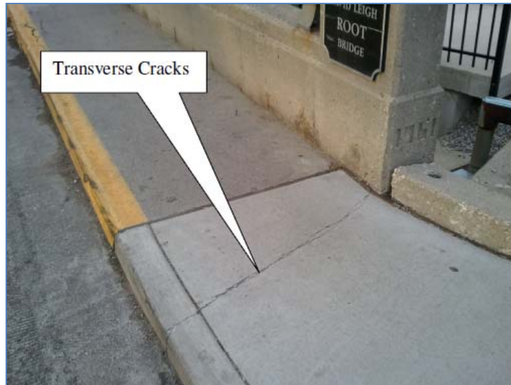
Figure 4. Transverse Cracking 5
