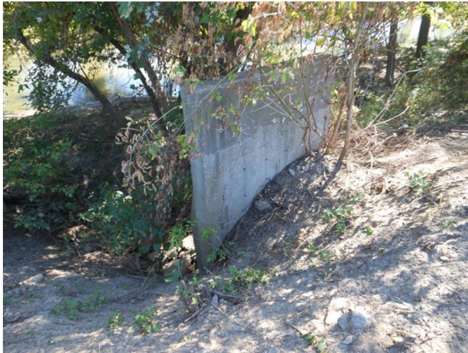
Figure 9 – Erosion around Headwall #3
