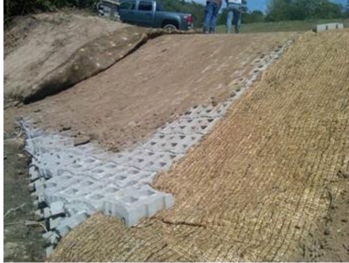
Figure 40- Open-Celled Articulating Concrete Block
