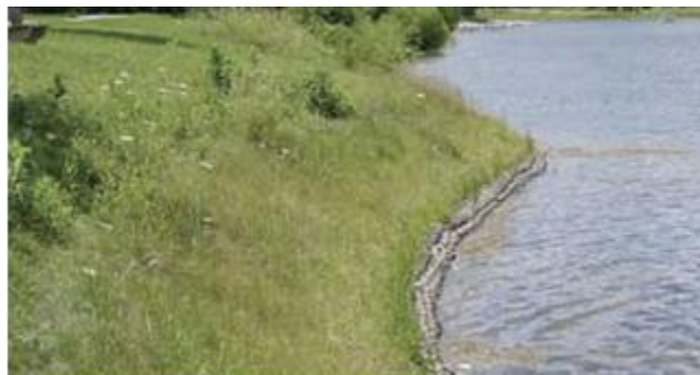
Figure 32 – Open-celled Blocks After Established Vegetation
