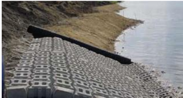
Figure 32 – Open-celled Blocks After Established Vegetation
