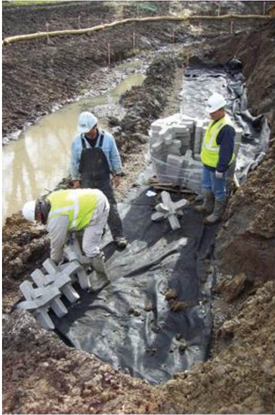
Figure 20 – Installation of A-Jacks
