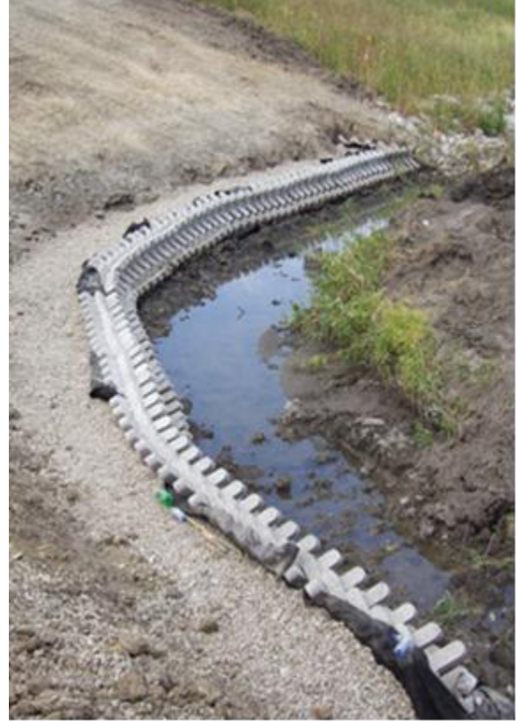
Figure 21 – A-Jacks along Channel
