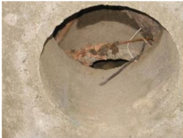
Figure 12- Erosion around Outfall #4
