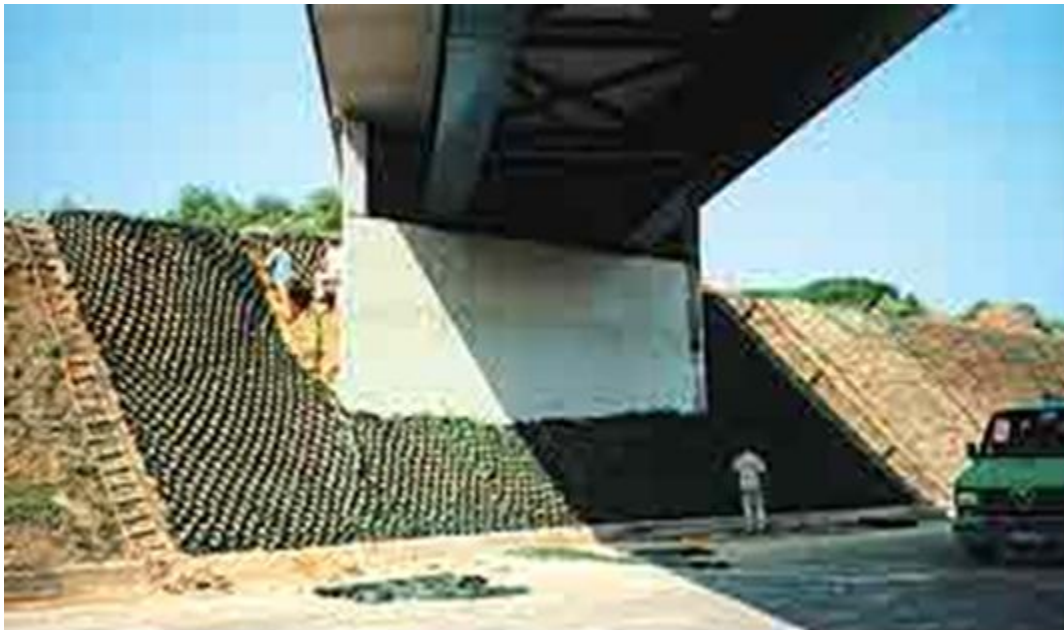
Figure 41- Installation of Geo-Mat
