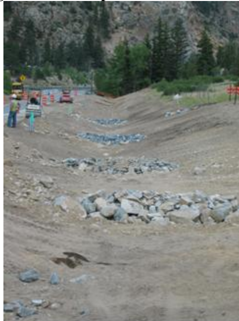
Figure 16 – Example of Rock Check Dams
