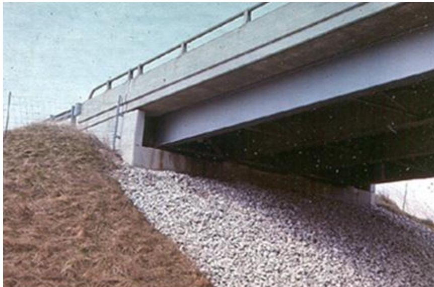
Figure 38- Application of Rip Rap
