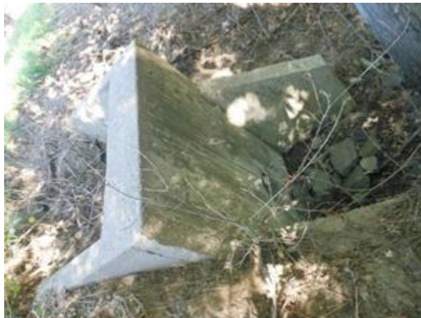
Figure 12- Erosion around Outfall #4
