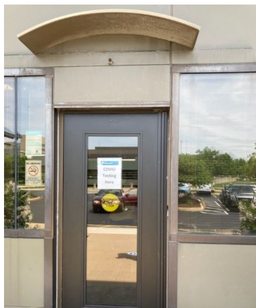
Covid Testing to the Right of Main Door
