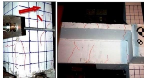
Vertical and Inclined Cracks at First-story Middle Column Base
