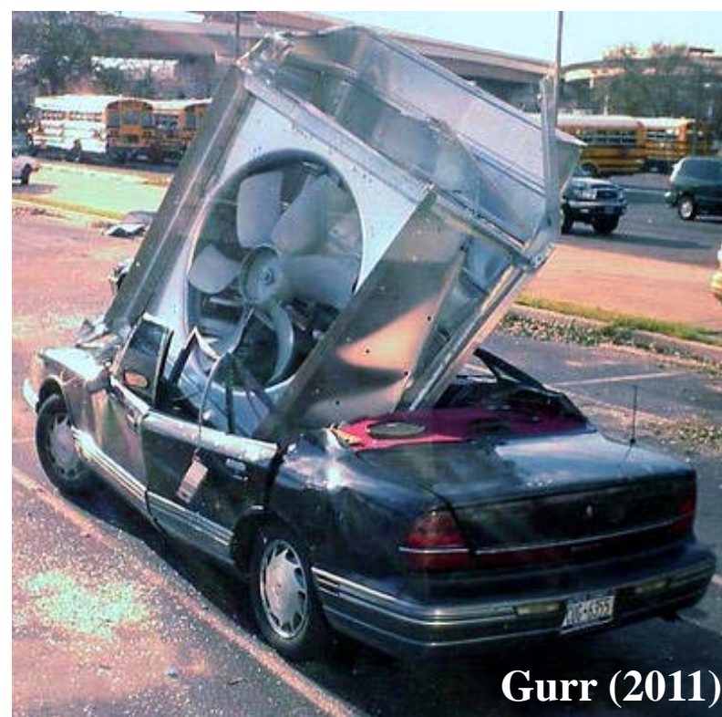
Fig. 1: HVAC anchorage failure.
