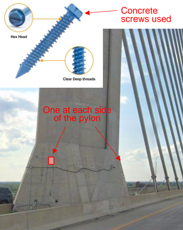
(c) External logger-radiation shield bundle installation locations (B side is shown)
