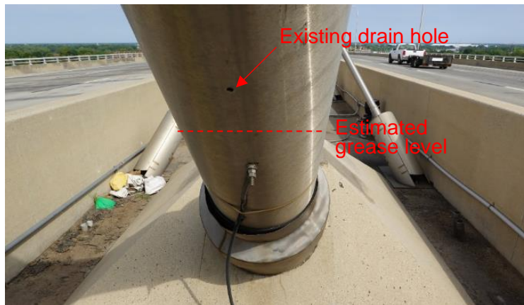
Figure 5 Lower ends of stays with a drain hole.
