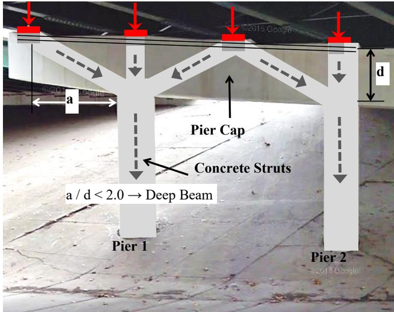
**Figure 1-1:** A sample pier cap
