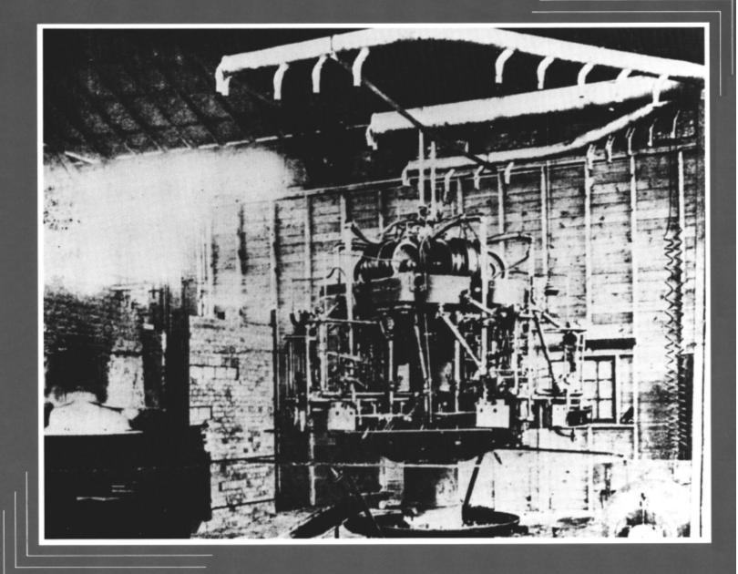
Also designed and built in 1912 was the original "AR" machine. Generally, it was an enlargement of the "AN," adapted to manufacture bottles of greater weight and capacity than prescription ware, such as beer and catsup bottles. It had an average production of 50,400 bottles per day.
