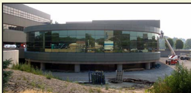
Construction on the new center will be completed next month.
