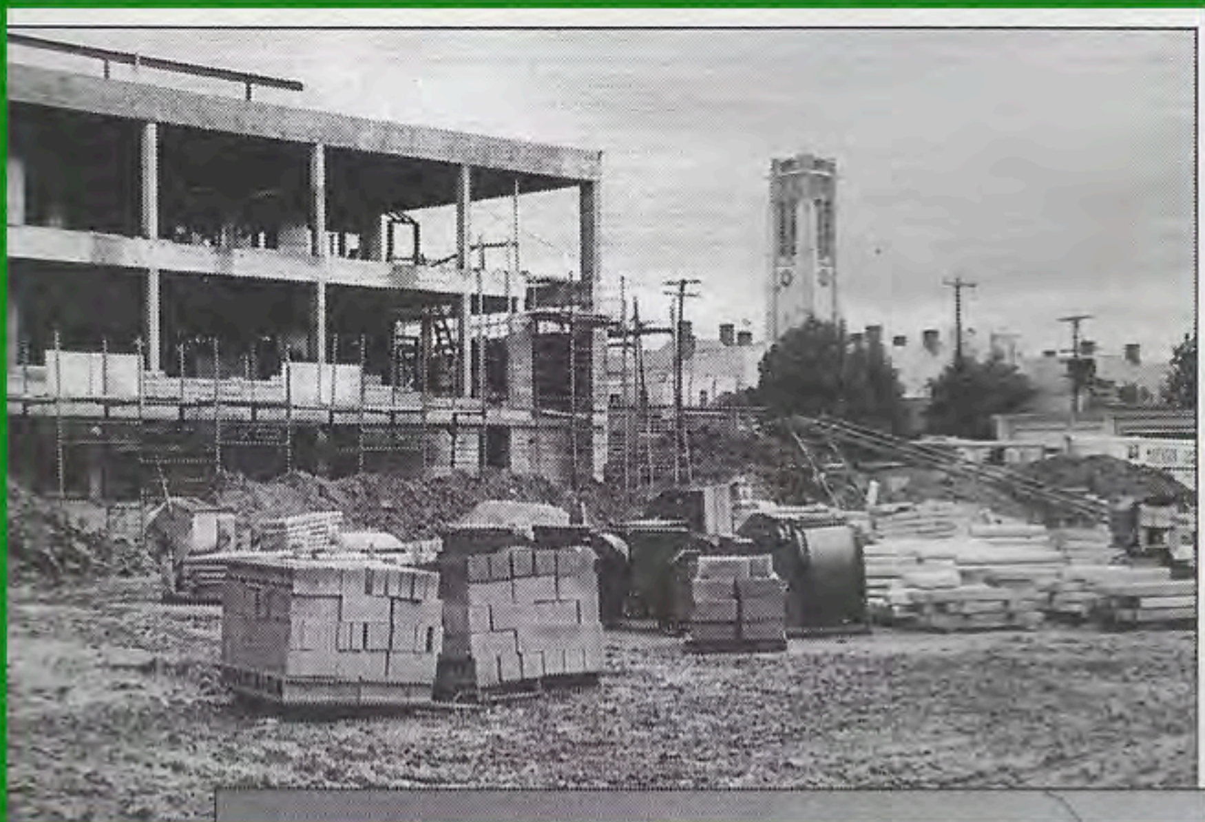
1966 Bowman Oddy Labs Construction
