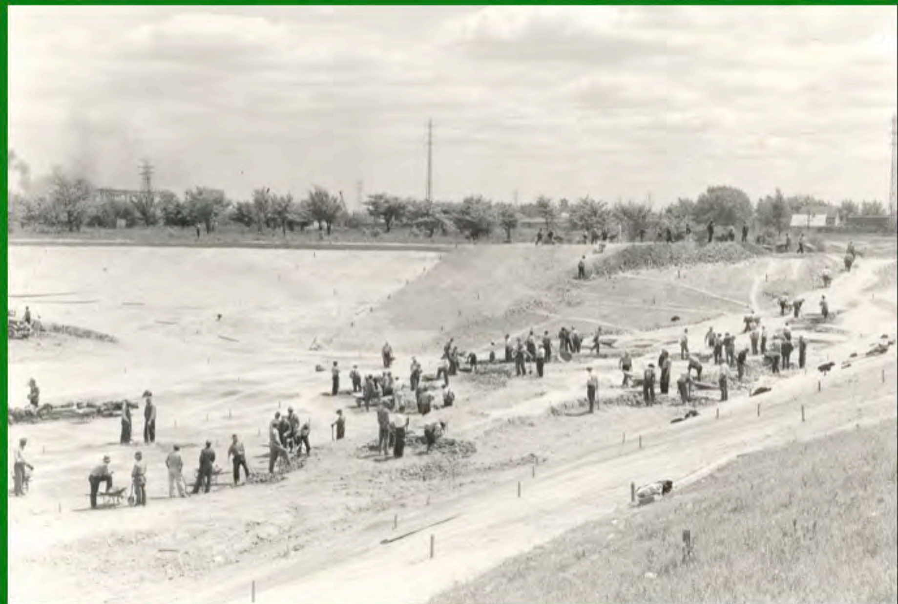
1922 Science Building Construction
