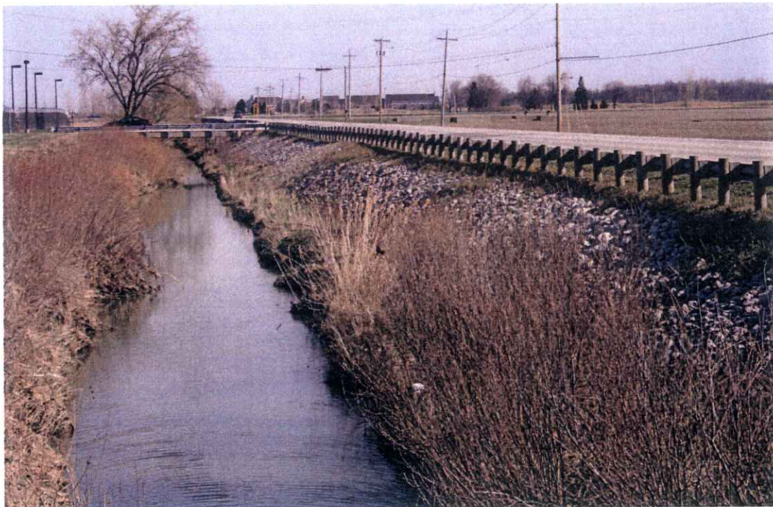
PHOTO 2: Berger Ditch at Field Site 2: surveyed reach adjacent to Oregon WTP.
