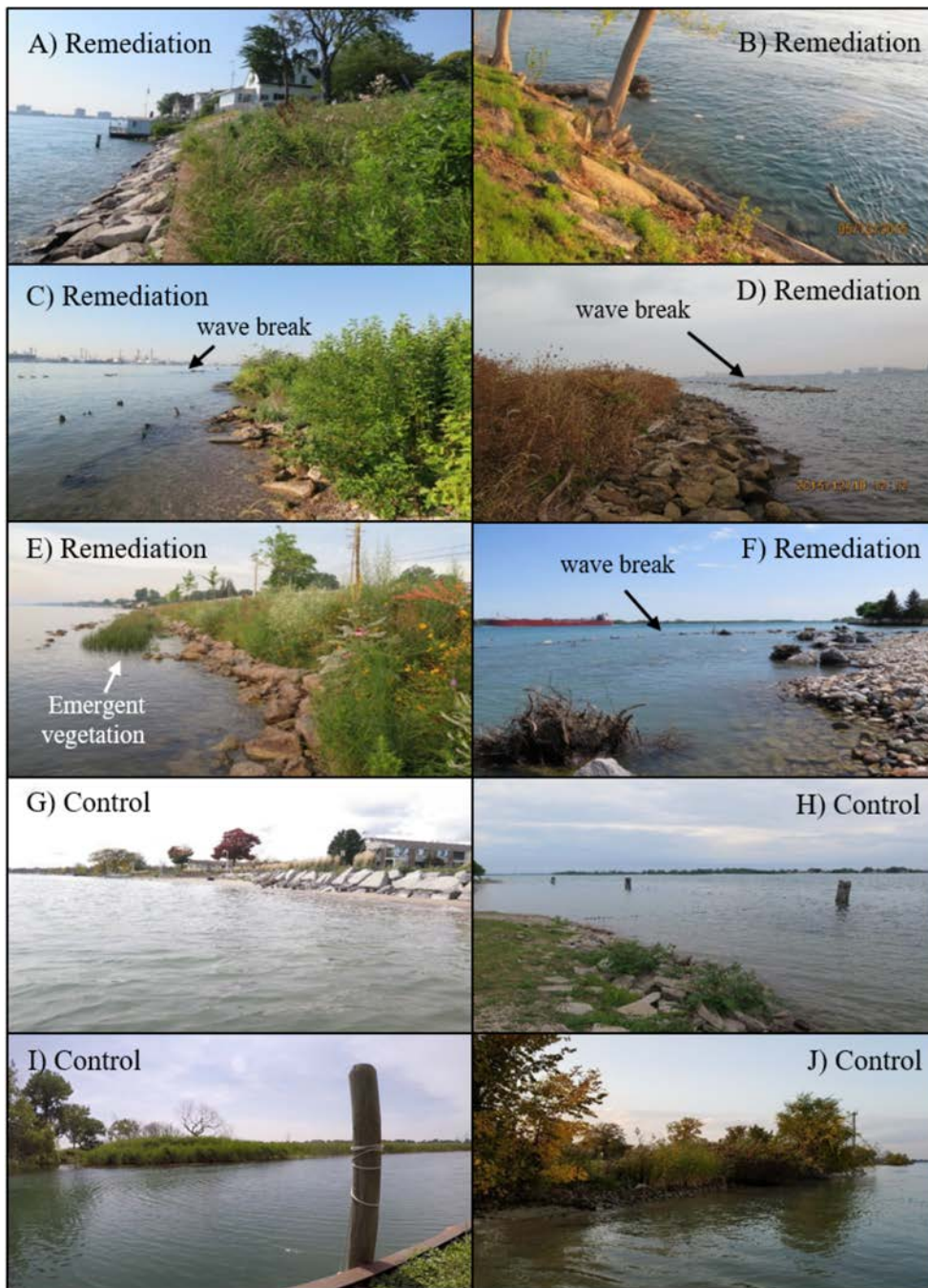
Fig. 2. Shoreline sampling sites in the St. Clair River. The Port Huron North (A), Port Huron South (B), Blue Water River Walk (C and D), Marysville Living Shoreline (E), and Cottrellville (F) remediation sites included a mixture of shoreline softening (e.g., removal of seawall), native vegetation, and placement of cobble, root wads, and boulders to provide in-stream structure. The top of wave breaks at the Blue Water River Walk (C and D) and Cottrellville (F) sites are highlighted with an arrow in the upper portion of each panel and a bed of emergent vegetation planted at the Marysville Living Shoreline is shown in panel E. In contrast, in-stream structure at the Marysville (G), Marine City Beach (H), and Algonac State Park (J) control sites was primarily limited rip-rap along the banks, although terrestrial vegetation over-hung portions of the bank at the Algonac State Park site and aquatic vegetation was prevalent at the Anchor Bay site (I).
