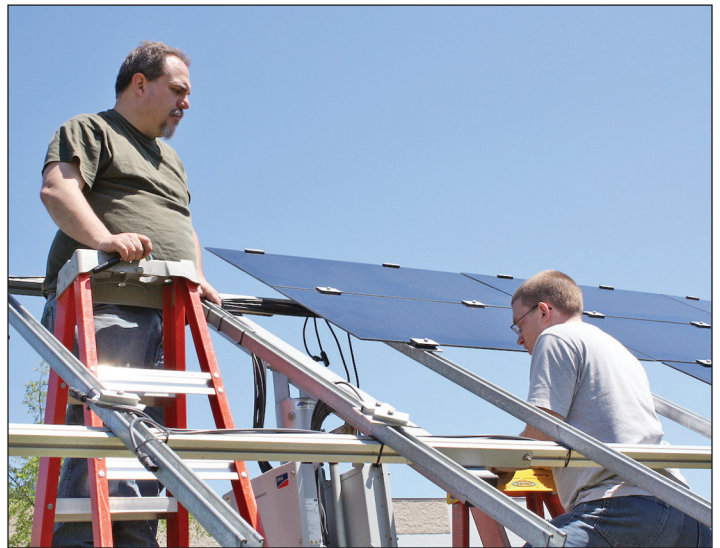
Undergraduate student David Raker and graduate student Paul Roland replace damaged modules to repair UT's 32 kW CdTe PV array.
