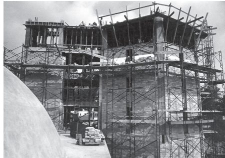
Construction of the Ritter Astrophysical Research Building.
