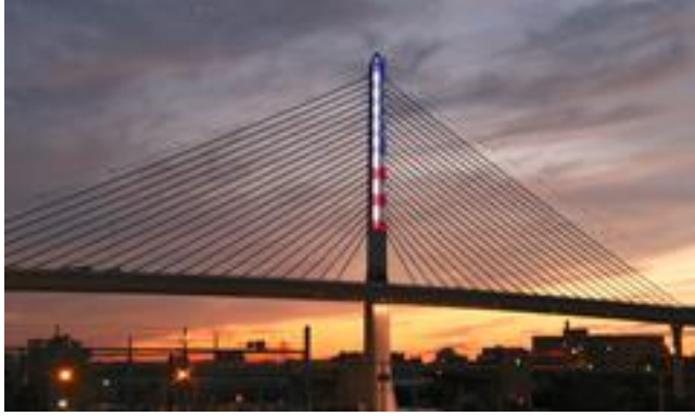
The pylon in the center of the Veterans' Glass City Skyway bridge over the Maumee River in Toledo, Ohio will be lighted with electricity from solar arrays in the highway right of way
