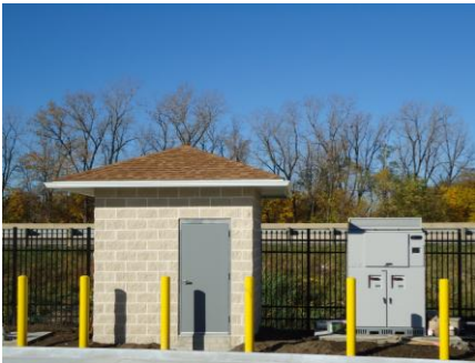
Building at the array site to house instrumentation for the solar research project.
